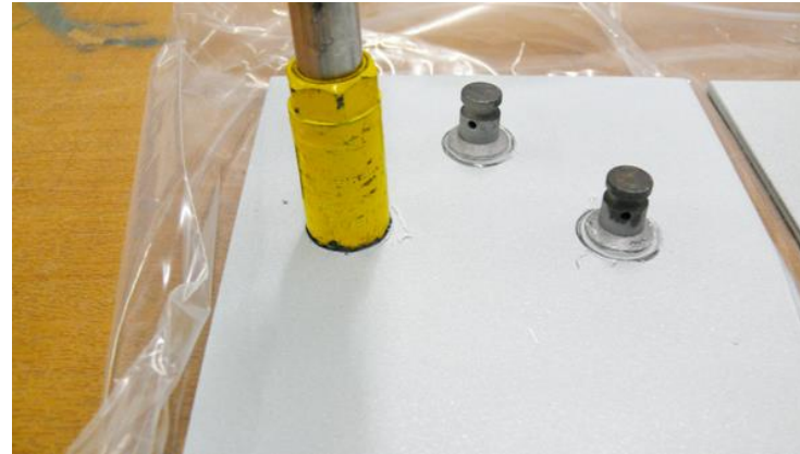
Bonding of test pieces and cutting free of glue and coating.
